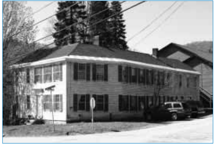
The Tontine apartment building is located at the corner of Guilford Center Road and Route 5, and is one building of three now owned by the Friends of Algiers, Inc.
